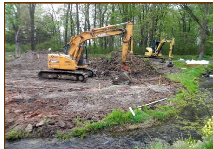
Construction: remove sediment, stabilize stream banks, create wetlands, establish native plantings
