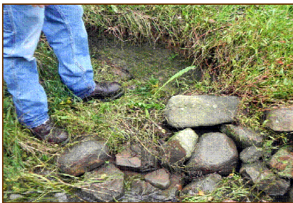
Pre-construction Conditions: erosion, bank slumping, flooding on golf course
