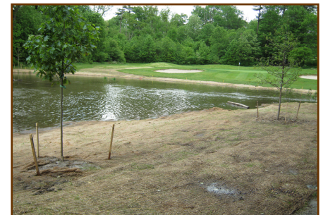
Completed Condition: vegetation is establishing, project survived first flood, increased wildlife activity seen
